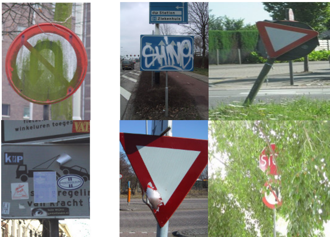
Figure 1: Examples of damaged traffic signs.
